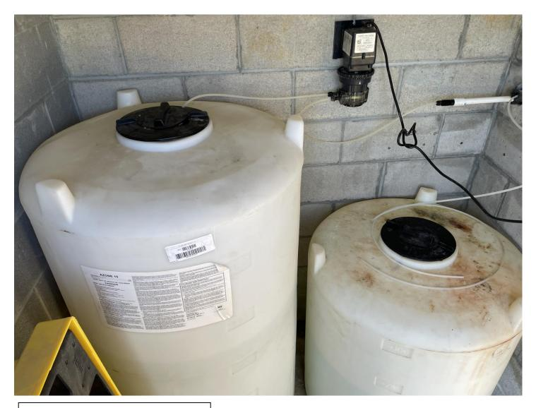
County Name: Bulloch Site Name: Brooklet Picture No. 6 of 6 Date: 12/19/2023 Weather: clear sunny Time: 12:31 PM Photographer: Lowery Program: DW Explanation: chlorination tanks at treatment plant 102
