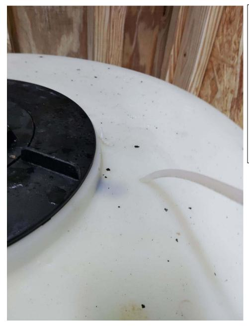
County Name: Bulloch Site Name: Brooklet Picture No. 7 of 9 Date: 2/1/2024 Weather: na Time: 8:11AM Photographer: Darrell Smith Program: DW Explanation: Lid screwed on with hole in container for chlorine line
