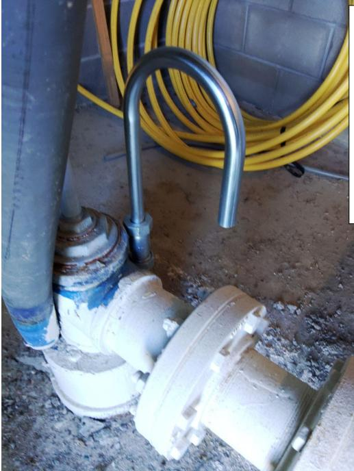
County Name: Bulloch Site Name: Brooklet Picture No. 9 of 9 Date: 2/1/2024 Weather: na Time: 8:40AM Photographer: Darrell Smith Program: DW Explanation: Installed riser pipe on source 102(well#2)
